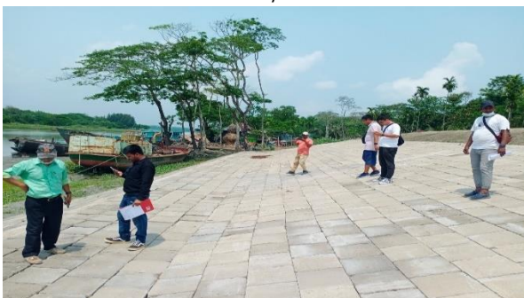
Figure 3-35: Closure across the Hetalia Khal (DS-11) of Polder-48
