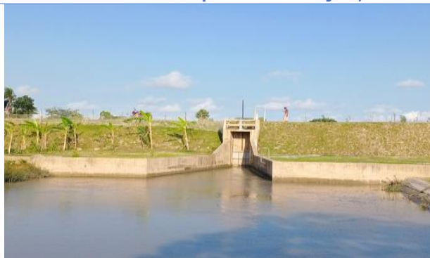
Figure 3-32: Complete Drainage Sluice DS-1 in Polder-40/2
