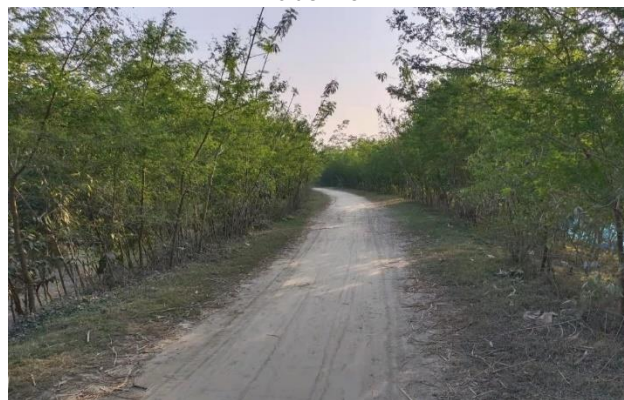
Figure 3-37: Completed Embankment of Polder-40/2
