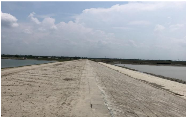
Figure 3-12: Nalian Closure Dam of Polder-32
