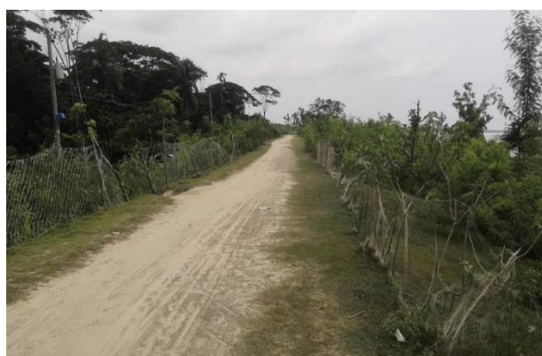
Figure 3-30: Turfing work for k13+100-k15+000 in Polder-40/2
