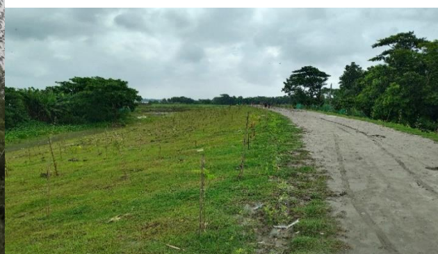
Figure 3-31: Turfing work for k12+000-14+000 in Polder-43/2C
