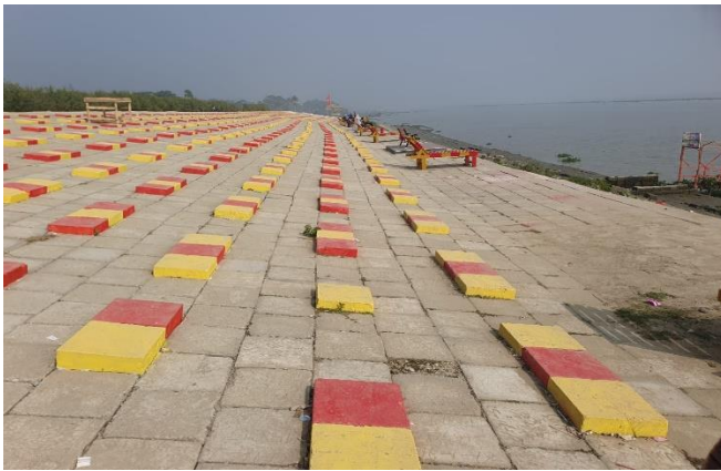
Figure 3-11: Completed Slope Protection Works in Polder-35/1
