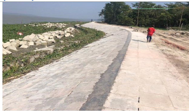
Figure 3-33: Slope & Bank Protection work in Polder-39/2C
